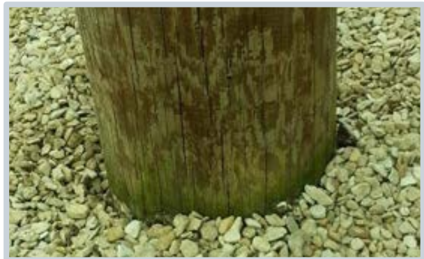
Initial visual inspection would suggest no problems with this pole
